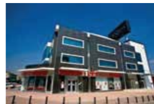
Location_Turkey Project_Office Building
