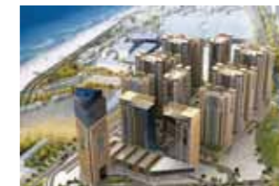
Location_U.A.E Project_Residential Building
