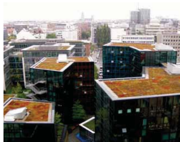
Location_Germany Project_Business Park
