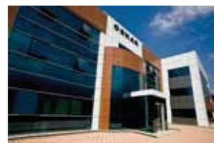
Location_Turkey Project_Office building
